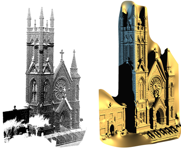
Fig. 3. LIDAR scan and smoothest restricted range reconstruction of St Marys church, LA. Foreground trees create occlusions in this scan.
